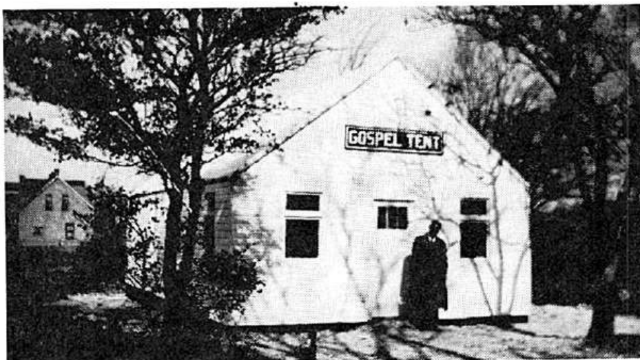
Portable Hall, Upper Prince Street, Charlottetown, 1941
