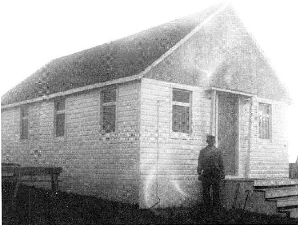
ERECTING OLD PORTABLE HALL
